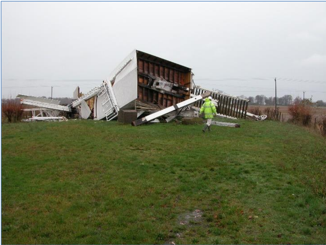
Figure 5 Chillenden windmill, blown down in 2003, now re-built
